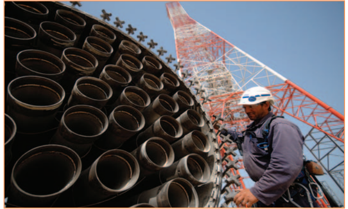
Inspecting the Qatargas 2 flare tip
