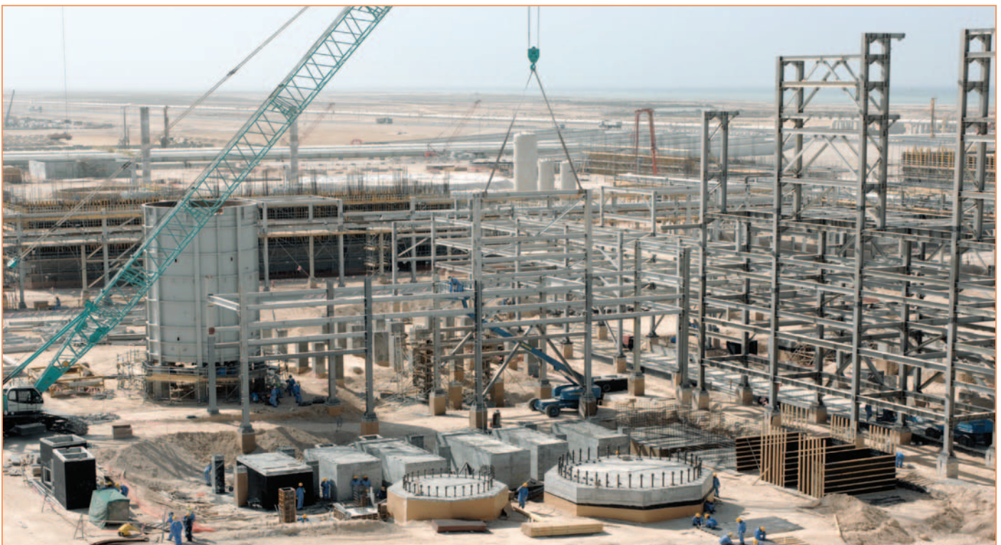
Aerial view of refinery piperacks
